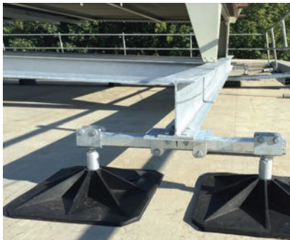
▲ Typical support utilising Flexi Twin Frames.
