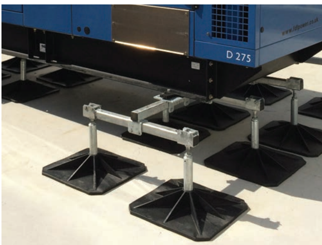
▲ Typical air handling unit support utilising Flexi Quad Frames.
