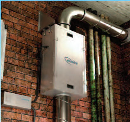
INSTALL IN ANY ORIENTATION WITH UMBILICAL KIT*
