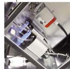
Figure I1g: Condensate pumps and bypass actuator where fitted.
