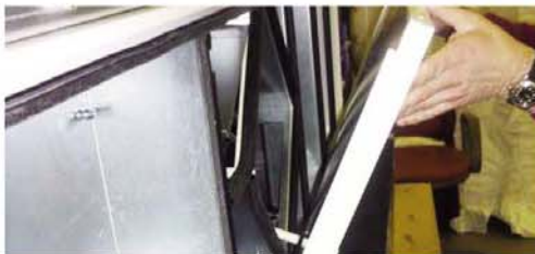
Figure I1a, I1b and I1c: Remove non control centre side access panel by removing the four bolts (2 x 2) on rear of panel and disconnect condensate pipe.
