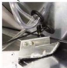
Figure I1f: Condensate intake position where fitted.
