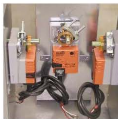
Figure I3a: Actuators are removed in sequence from accessibility.
